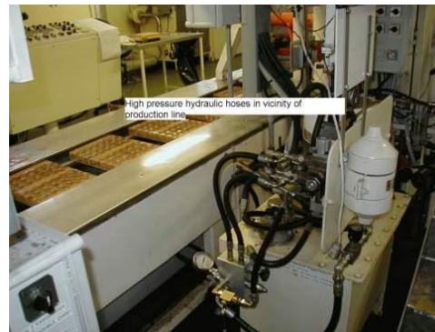
Hydraulic hoses near foodstuff
